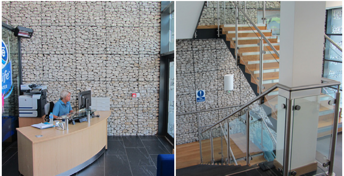
As these photos illustrate, the exterior and interior walls of the Nestlé Waters building show the success with which architectural features can be emphasised—using a combination of gabion mesh systems supplied by Enviromesh—and carefully specified aggregate/filling material
