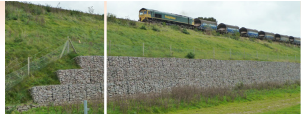
Completed works at the Sharnbrook rail embankment project, Bedfordshire
